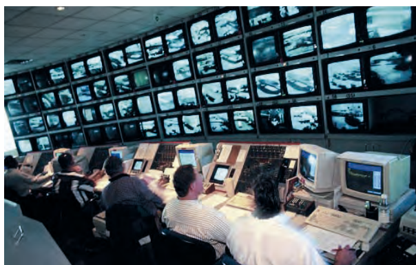
Fig. 1: Outdated CCTV-Surveillance system using the sensor monitoring concept.
